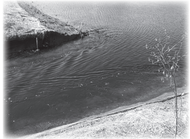
New inlet through dyke allowing tidal flooding of salt marsh plants.
