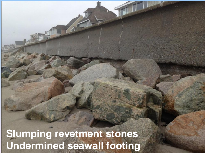
Exposed seawall toe Exposed rebar
