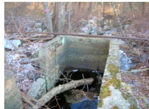
Mill Pond Dam in disrepair
