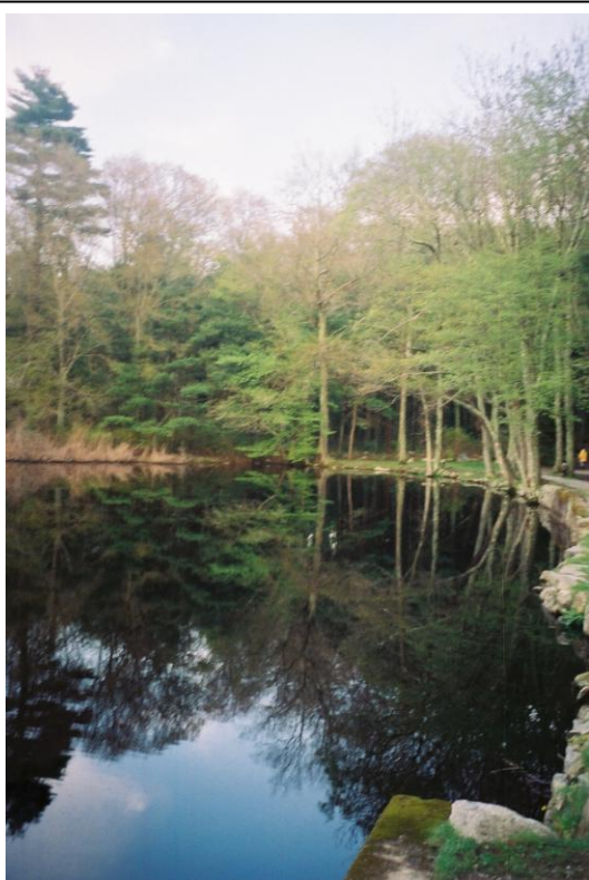
A dam on Second Herring Brook at Norris Reservation in Norwell. The pond is located in a conservation area. It provides a nice view alongside the walking path and benches in the upper right hand side of the photo. People might not want to see this pond disappear at this location even though it would improve habitat for native and migratory species.
