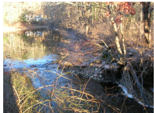
Mill Pond Breached Dam
