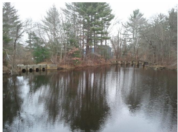
The dam that forms Forge Pond at King Street on the Drinkwater River upstream of the Indian Head River in Hanover still exists today.
