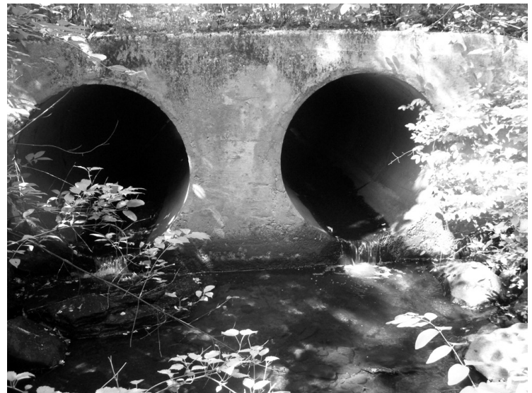
Culverts on Iron Mine Brook to be removed this fall.
