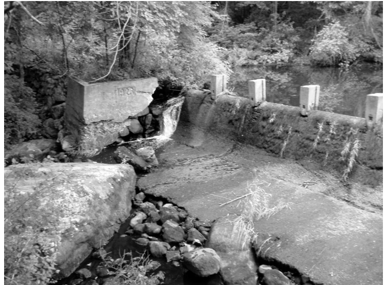
Tack Factory Dam to be removed this fall on Third Herring Brook.
