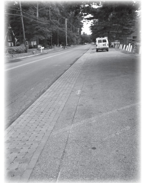
Permeable pavers on Washington Street in Pembroke
