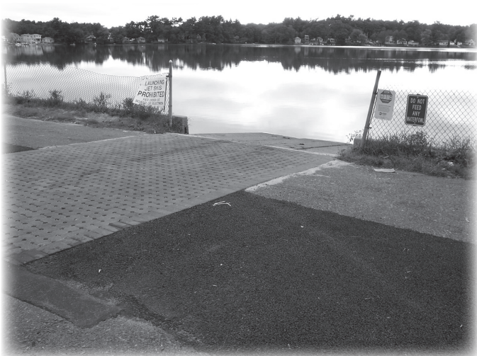
Porous pavement and permeable pavers at Oldham Pond Boat Ramp in Pembroke.
