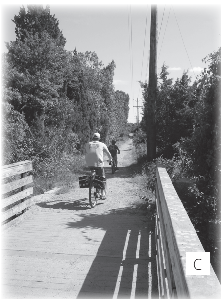
A view of the bike trail/bridle path at the Francis Keville Memorial Bridge.
