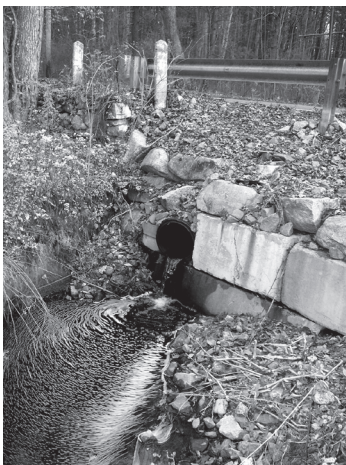
Culvert in Furnace Brook, Marshfield - Example of Fish and Flow Barrier
