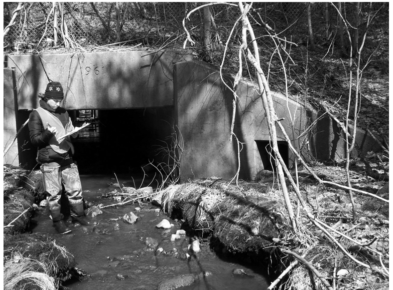
NSRWA Volunteer of the Year Sara Frazier assessing culverts for fish passage
