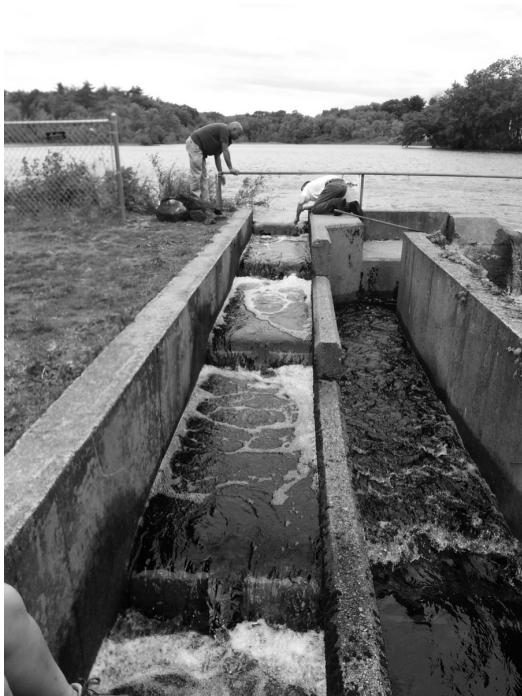
First Herring Brook/Oak Oaken Bucket Pond fish ladder with new weirs.
