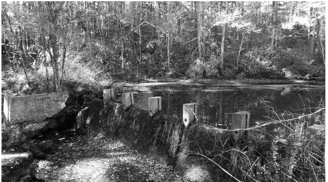
Tack Factory Pond Dam in Hanover - September 2013
