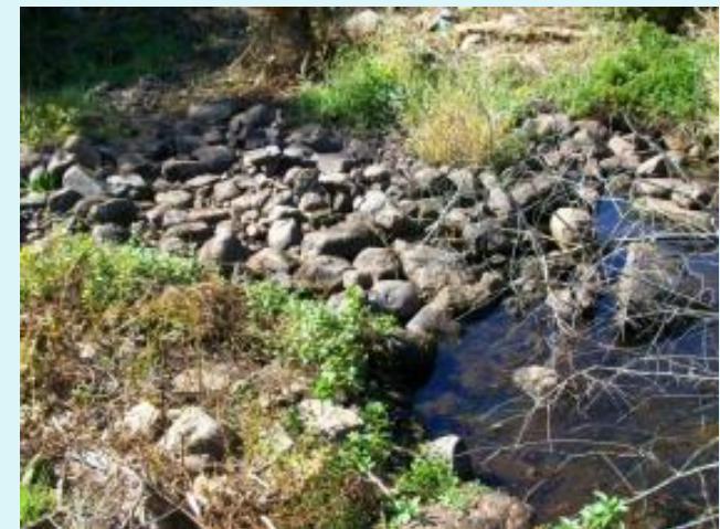
Entrance channel improvements
