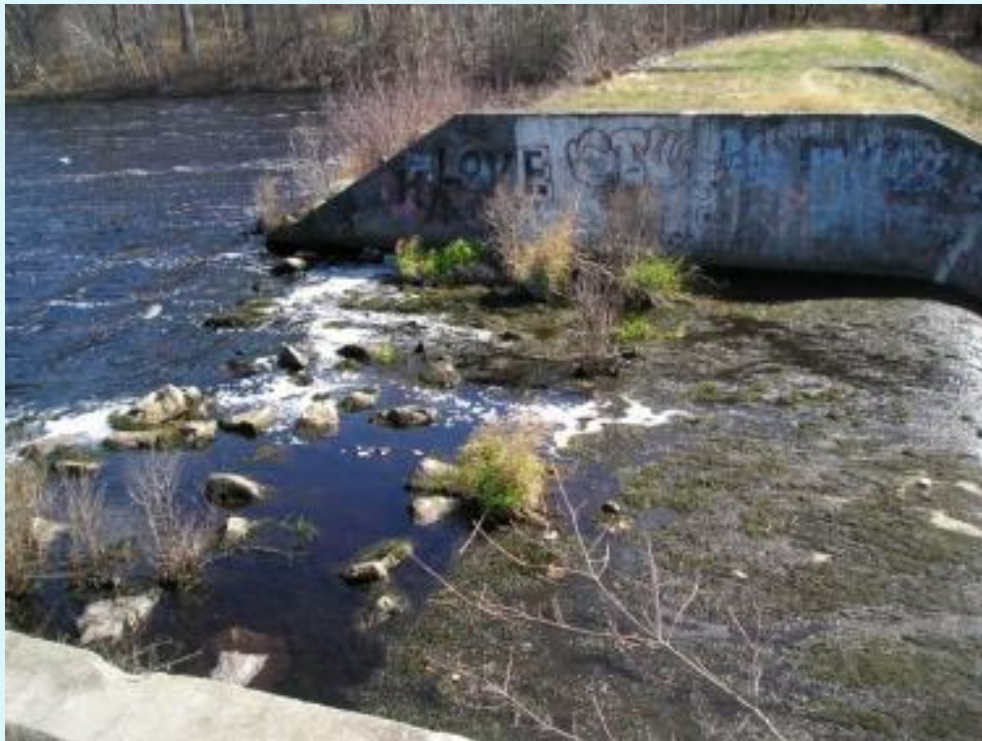
Lower Spillway Crest
