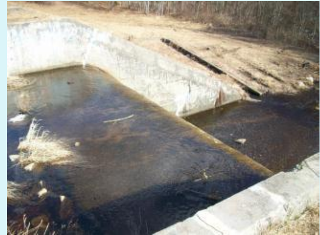
Spillway bottom hinged crest gate
