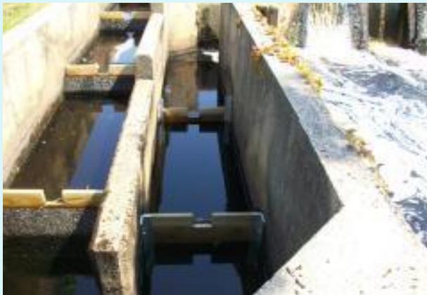
Fishway weir modifications
