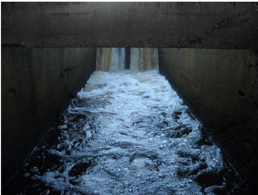
Photo 19B – Primary spillway discharge channel
