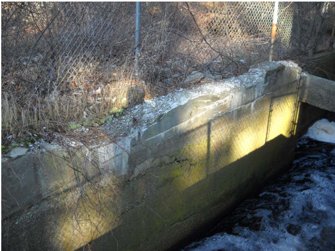
Photo 21A – Spalled concrete on left outlet channel wall
