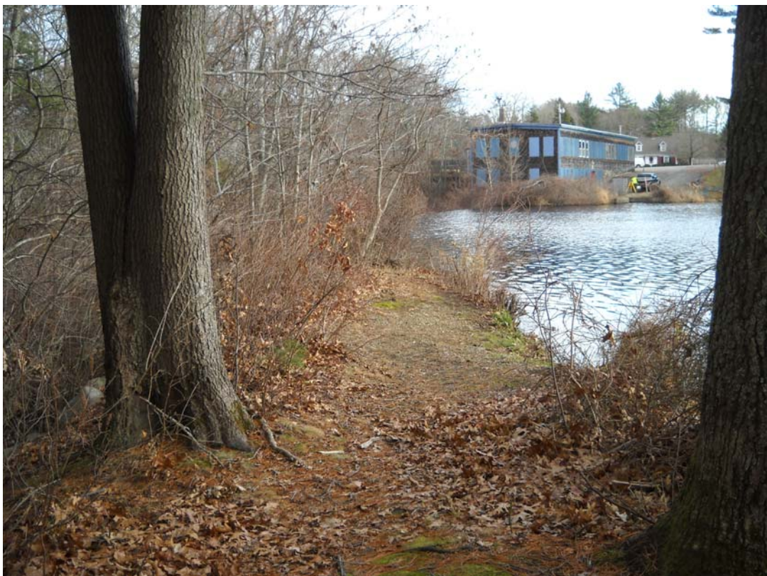
Photo 21V – Trees and brush on left embankment (from left abutment)
