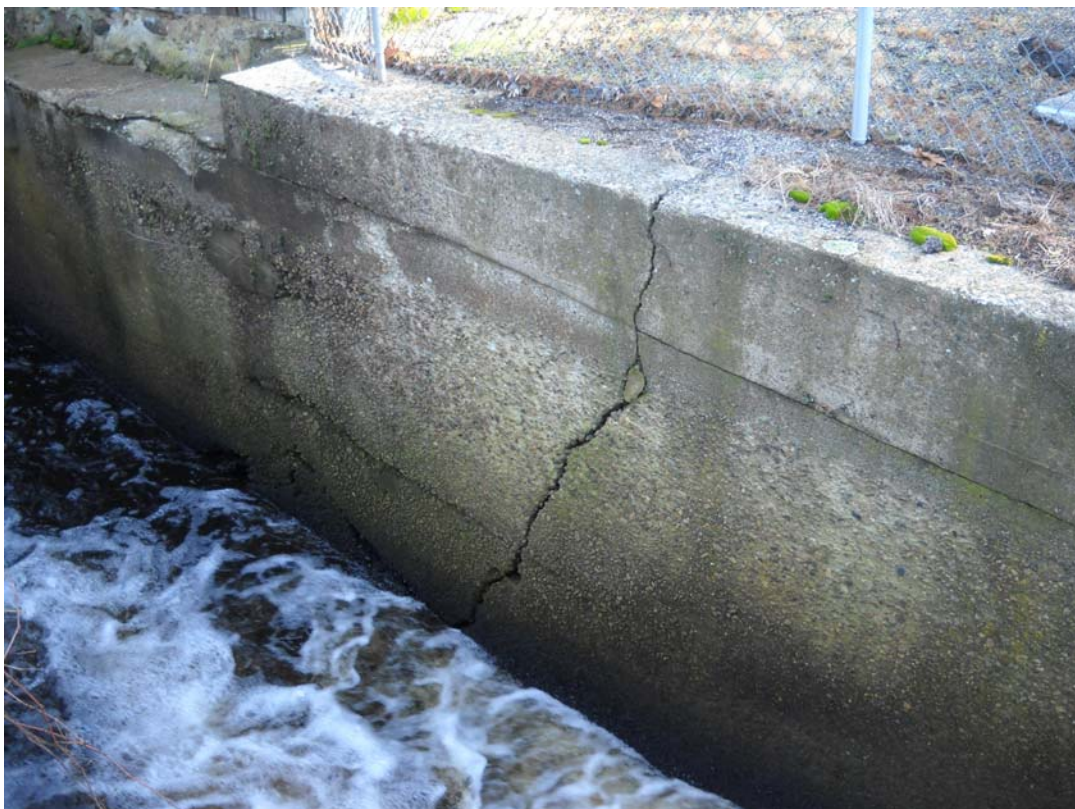
Photo 21C – Cracks in right outlet channel wall
