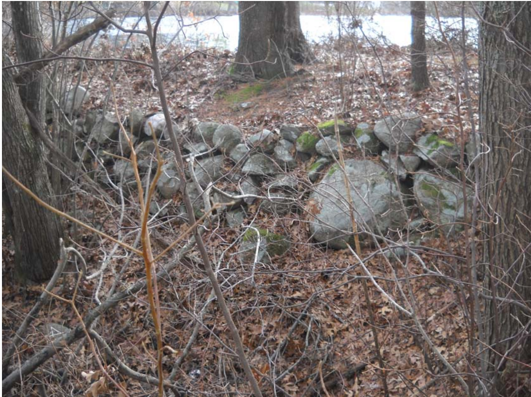
Photo 21W – Trees on crest of left embankment and adjacent to downstream vertical fieldstone masonry wall
