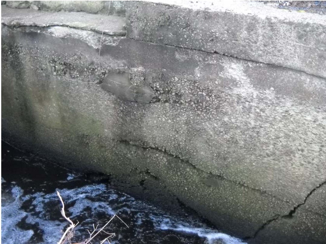
Photo 21D – Cracks in right outlet channel wall
