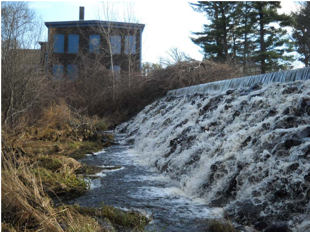
Photo 21S – Brush on embankment between spillways
