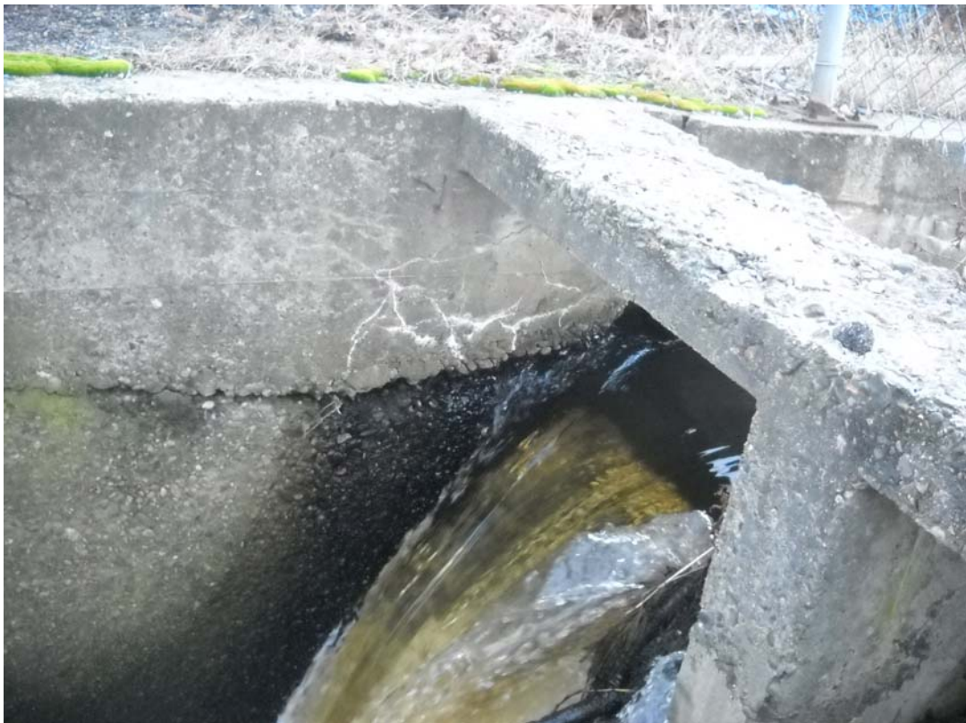
Photo 21E – Crack in wall at right of weir (note spalled concrete on beam)
