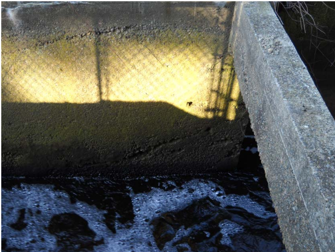
Photo 21B – Exposed aggregate/deteriorated concrete on left outlet channel wall
