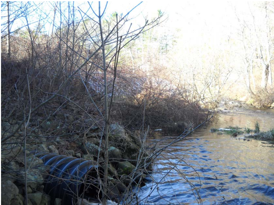
Photo 21R – Brush on embankment between spillways (from right abutment downstream)
