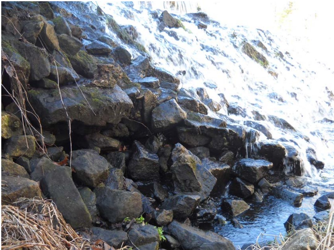
Photo 21G – Area of missing/fallen riprap at right auxiliary spillway contact
