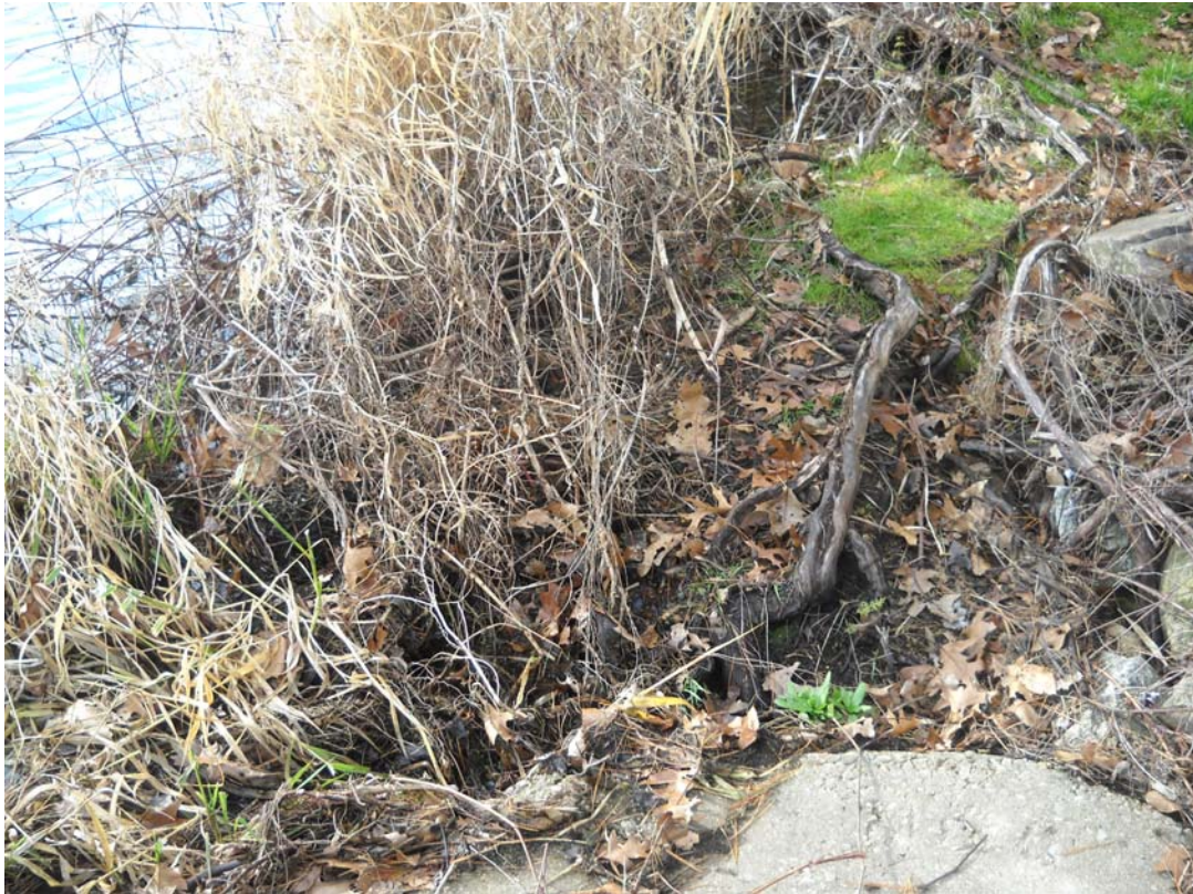
Photo 21L – Exposed roots, erosion and sinkholes upstream face and crest near left auxiliary spillway contact
