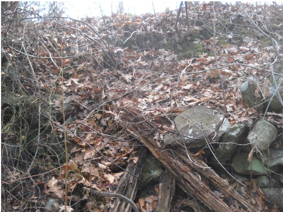
Photo 21K – Collapsed vertical wall approximately 50 feet from left abutment
