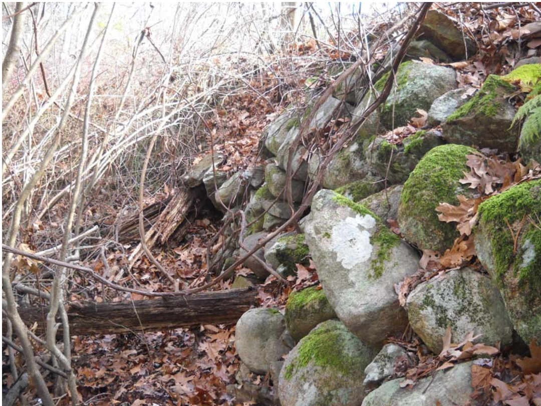
Photo 21J – Collapsed vertical wall approximately 50 feet from left abutment
