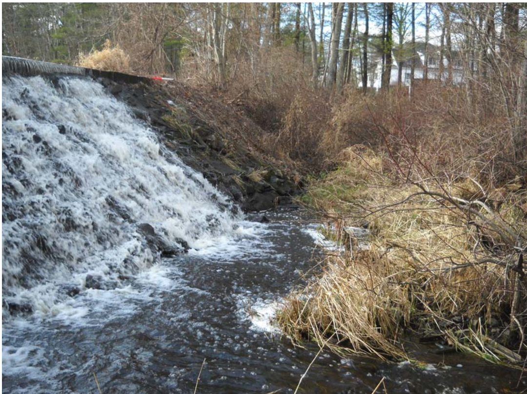
Photo 21T – Brush on left embankment
