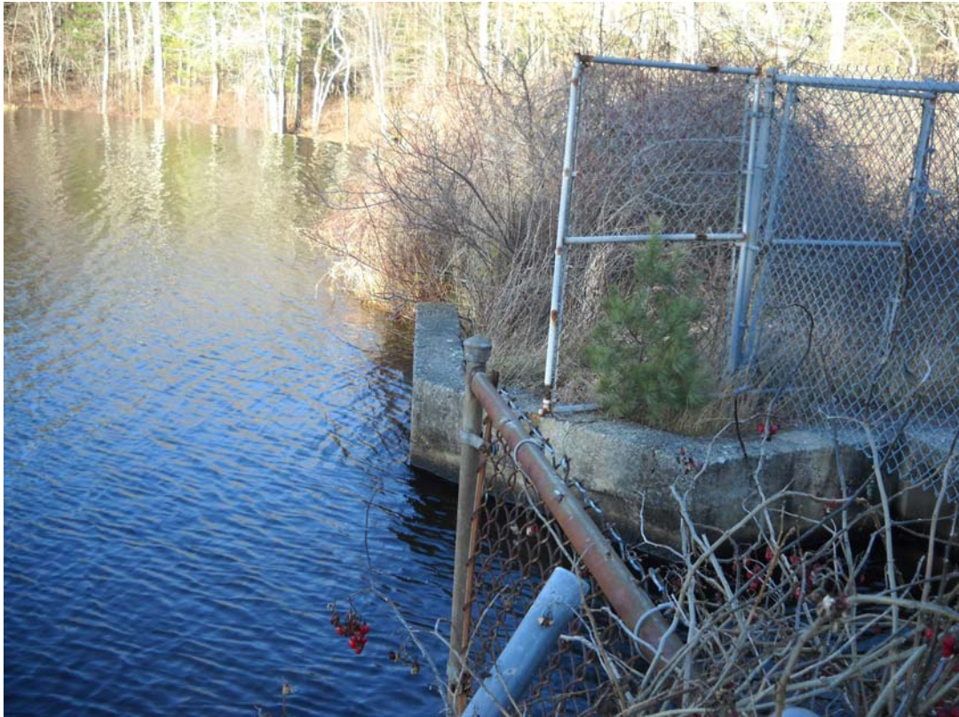
Photo 21Q – Brush on embankment between spillways (from right abutment upstream)
