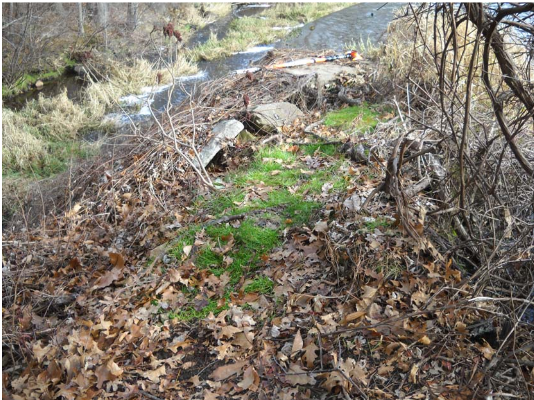
Photo 21M – Exposed roots and sinkholes downstream face and crest near left auxiliary spillway contact
